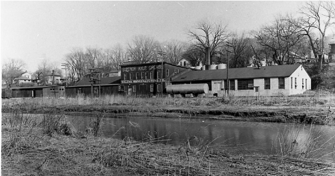
Figure 36. Galena Manufacturing buildings in 1946, as planning begins for levee construction. U.S. Army Corps of Engineers photo.
