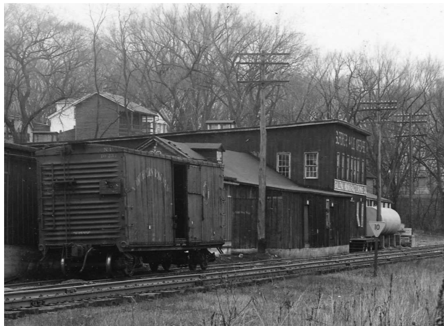
Figure 18. Galena Manufacturing looking southeast circa 1940s. Terry Miller
