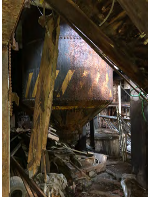
Figure 22. Axle Grease showing one of original tanks. Lower level looking northeast
