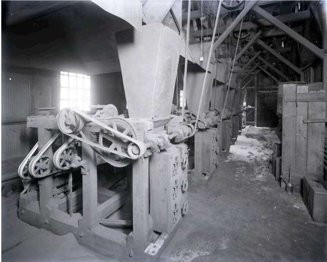
Figure 15. Axle Grease building interior showing mixing equipment, circa 1920s. Terry Miller, State Historic Sites Office.
