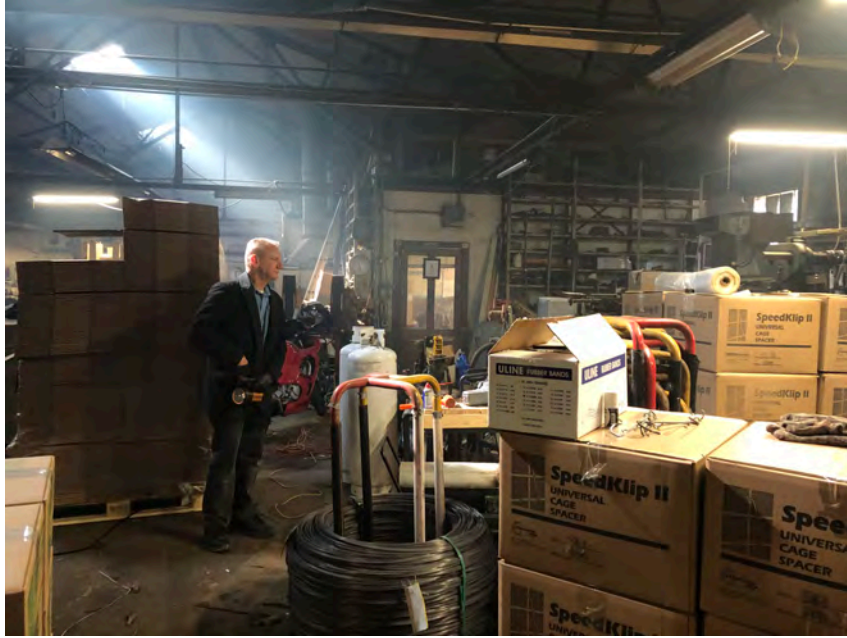
Figure 27. Axle Grease south addition where fabrication work continues as of 1.11.2023. Andy Willis in picture.
