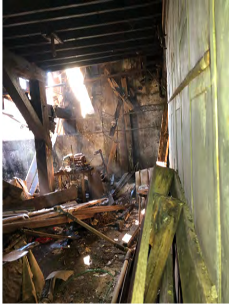
Figure 25. Axle Grease bldg. Southeast corner looking east. 1.11.2023.
