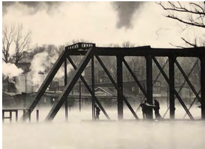
Figure 20. Flood of 1929 shows IL Central switch bridge in foreground and Galena Manufacturing in background. Reports of Floods in the Galena River Valley by Jeanne LeBron, 1937.
