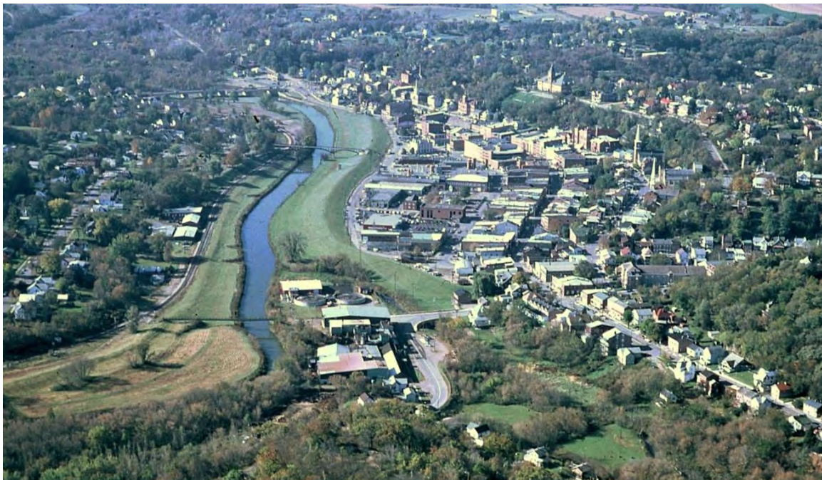
Figure 26. Galena Levee in the 1980s. Galena Manufacturing center left of image. Flood protection was complete for the west side of river but marginal for the east side.
