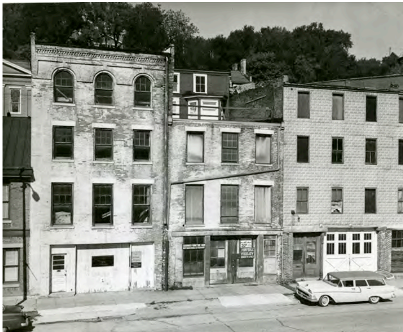
Figure 3. Middle bldg. (513 S. Main) was second location of Frazer's Galena factory, this from 1870 to 1883. Alfred Mueller Collection.
