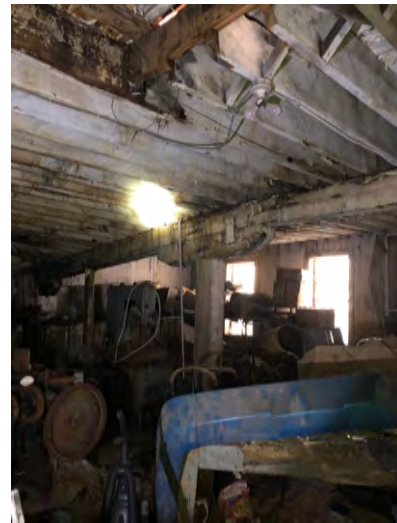
Figure 35. Axle Grease, first floor-looking southwest. Photo taken January, 2023.
