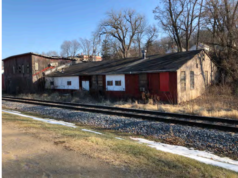
Figure 38. Galena Manufacturing looking northeast. Building on right is 1911 addition, still in use. Photo taken January, 2023.
