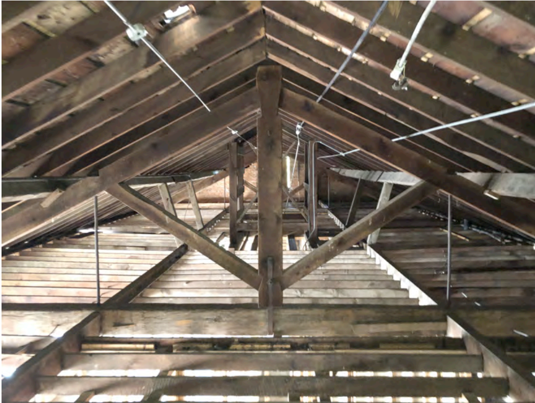
Figure 7. St. Mary's School showing roof truss system of 1864 section. Many downtown commercial buildings used this or similar construction, including area barns. Photo taken 14 September 2020.
