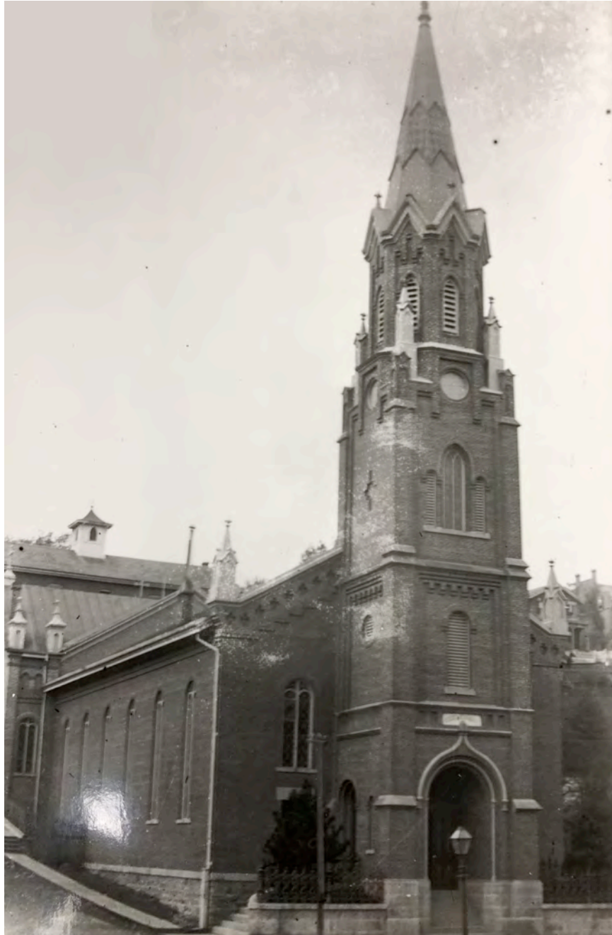
Figure 4. St. Mary's Catholic Church, circa 1880. Looking west from Franklin. The steeple was added in 1875-1876. The cupola in the upper left identifies St. Mary's School. Alfred W. Mueller Collection, Galena State Historic Sites Office.
