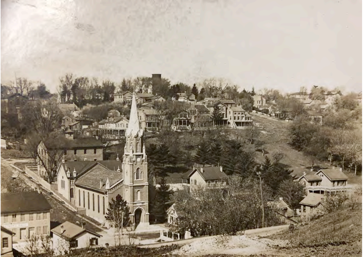
Figure 8. St. Mary's Catholic Church with its huge ornate steeple. The sanctuary is on back of the church with the school behind that (note cupola on school). Shreiner's Hall, a German community hall, is across Hill St. to the left and to the right of the church is the rectory. Alfred W. Mueller Collection - Galena State Historic Sites Office.
